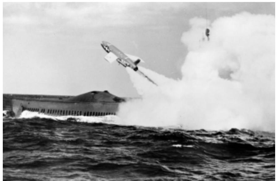
In the 1950s and 1960s, the Navy test-fired from submarines nearly 1,000 Regulus I cruise missiles, which were the size of contemporary fighters. This was the first shot from USS *Halibut*.
